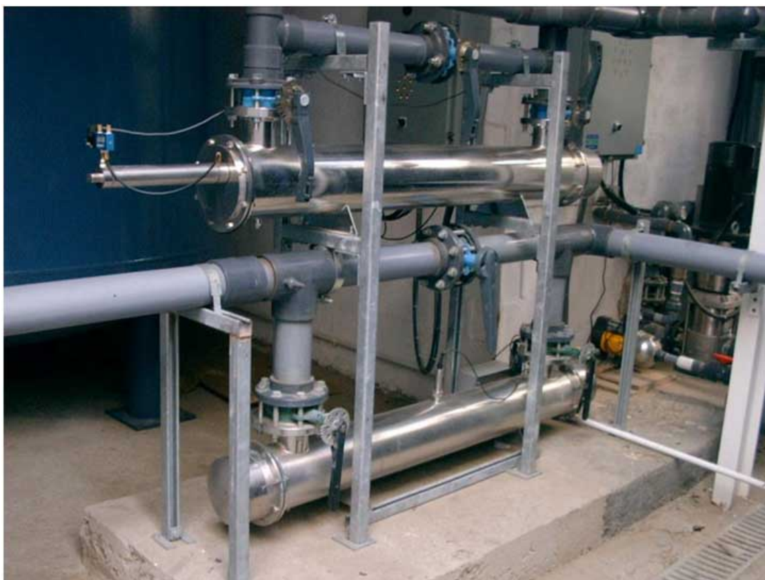
Monitoring Ultraviolet irradiation for deactivating bacteria in Zamzam water
