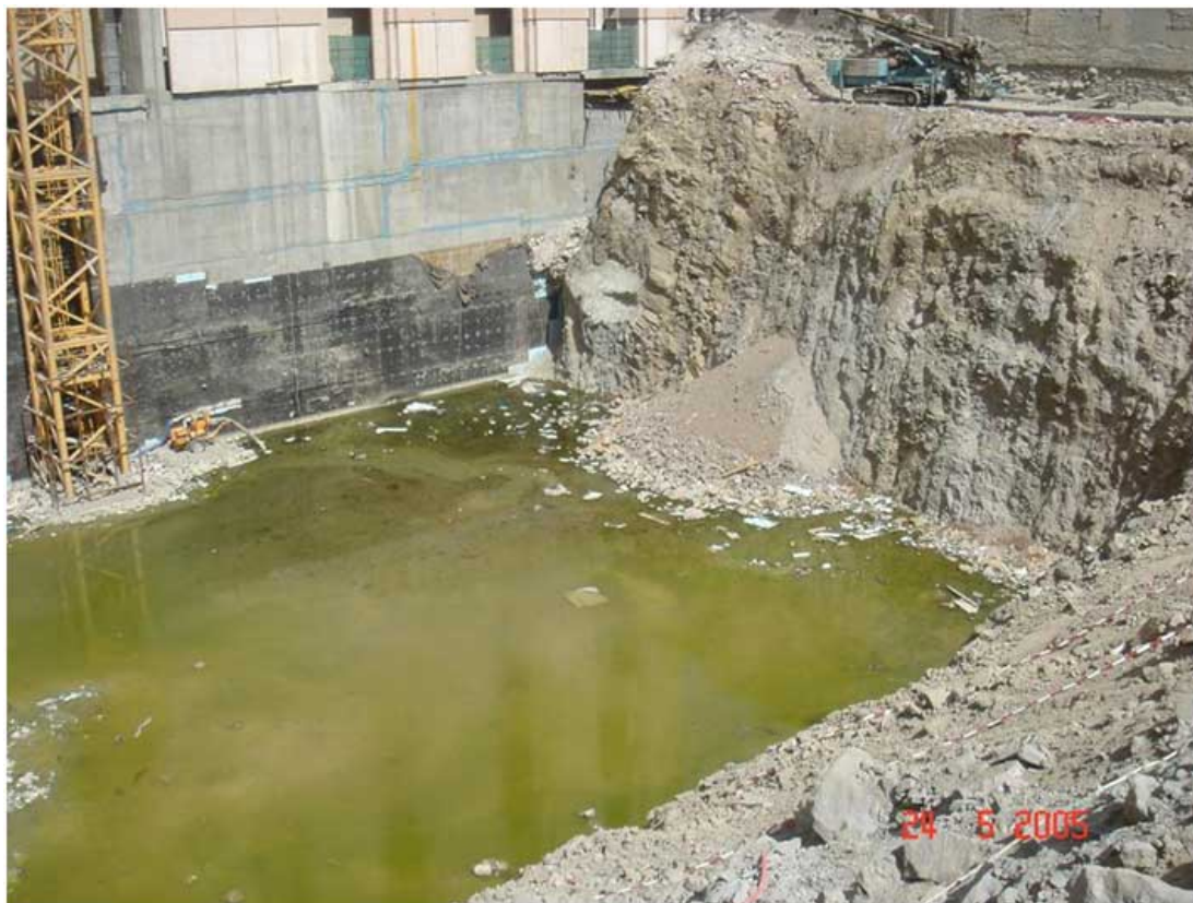
Excavation for foundation of King Abdulaziz Endowment Project
